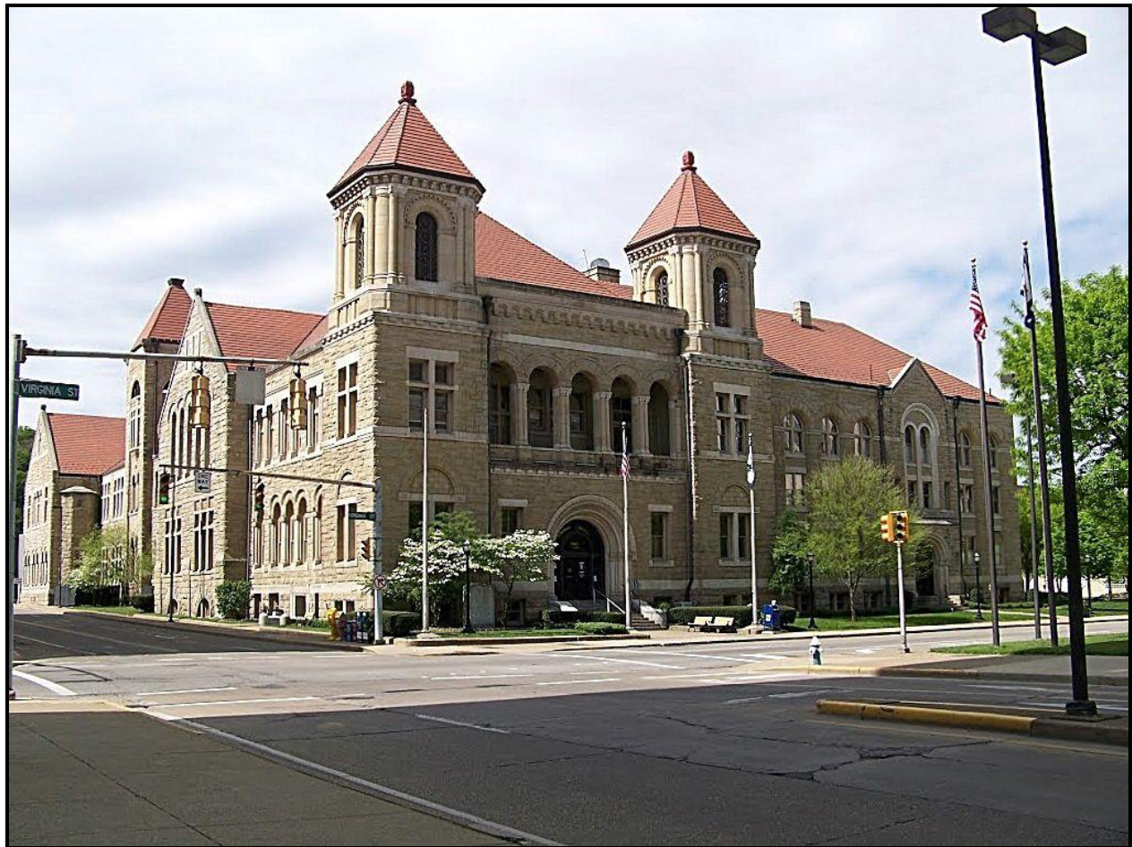
Kanawha County Courthouse
