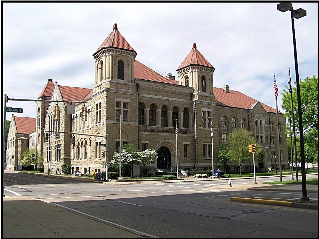
Kanawha County Courthouse
